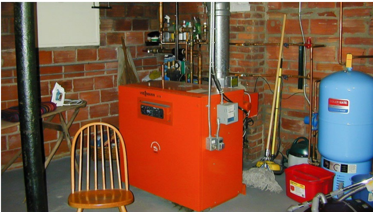
House we bought at 1921 Cambridge Road. Basement.
